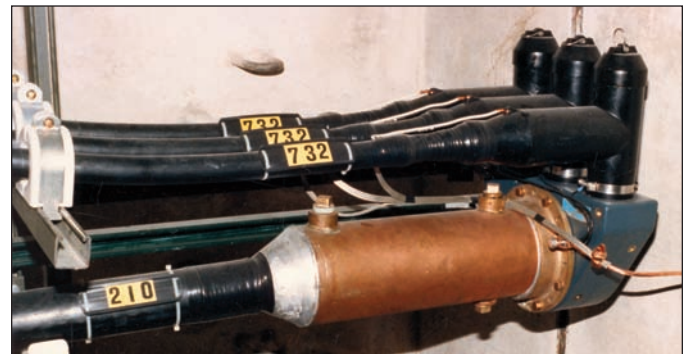
▲ G&W's 15/25kV deadend joint in a vault application.
