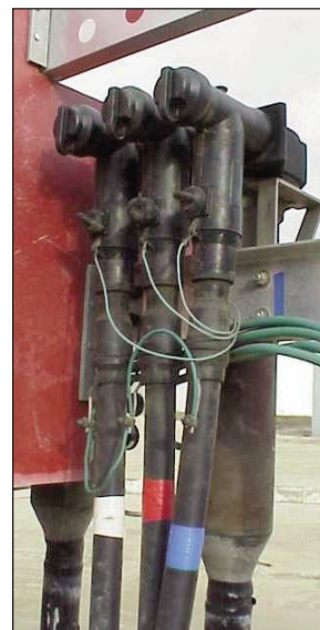
▲ G&W's 15/25kV deadend joint in a substation application.
