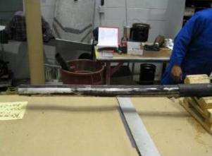
**3.5.5** Clean the aluminum sheath and slide over the cable the body assembly with copper sleeve facing towards cable end. Mark aluminum sheath per dimension 2 shown in the cable end preparation drawing and cut it straight. If the cable is fitted with a small bore gas carrying tube then this should be terminated 150mm in front of the sheath cut and formed vertically to avoid cable compound blockage. Exercise caution not to scratch or cut underlying cable cores.
