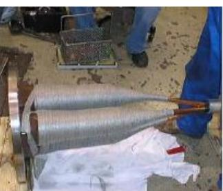
**3.7.6** Group all 3 braids and crimp them together in the provided crimp eye lug. Connect the lug to the earthing hole on the interface plate with provided earthing screw and lock washer.
