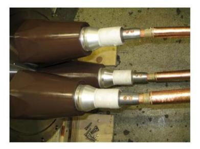
**3.6.2** Solder the conductors into the lugs. Exercise caution not to overheat cable insulation during this process. After the solder cools down polish the soldered surface to make it smooth. Make sure there are no protrusions or sharp edges. The transition from ferrule to cable conductor must be gradual and smooth without a step.
