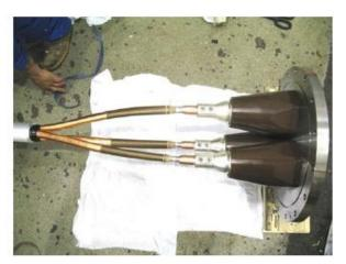
**3.6.6** Fill the bolt holes on the connectors and gap between the bushing and connector with provided epoxy filler putty. Clean the surfaces from excess of the putty with dry, lint-free cloth.
