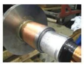
**3.8.2** Wire brush the exposed cable aluminum sheath and body copper sleeve for later application of the wiping sleeve between the two. Make sure surfaces are oil-free and clean from any contaminants.
