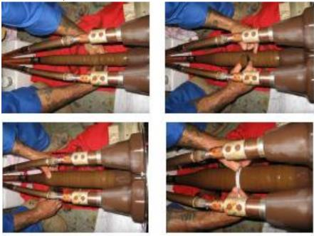
**3.7.3** Begin the ground electrode over the paper cone per Cable end preparation drawing by tightly applying one half-lapped layer of semi-con oil impregnated crepe paper tape. End the tape on cable copper tapes and secure from unraveling.
